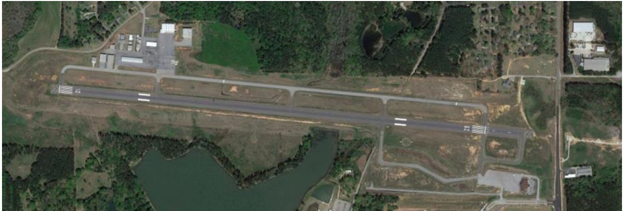
Figure 2-2: Covington Municipal Airport
